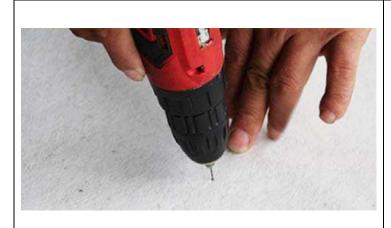
Use appropriately sized drill bits (0.75/1.0/1.5 mm) to drill holes on the roof.
